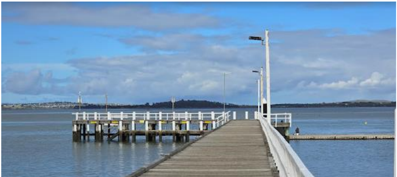
Photo 1: Rhyll Jetty - left arm fixed jetty head, right arm floating pontoon
