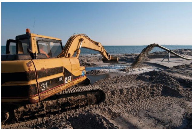
Above: Excavator moving piped dredged sand and slurry
